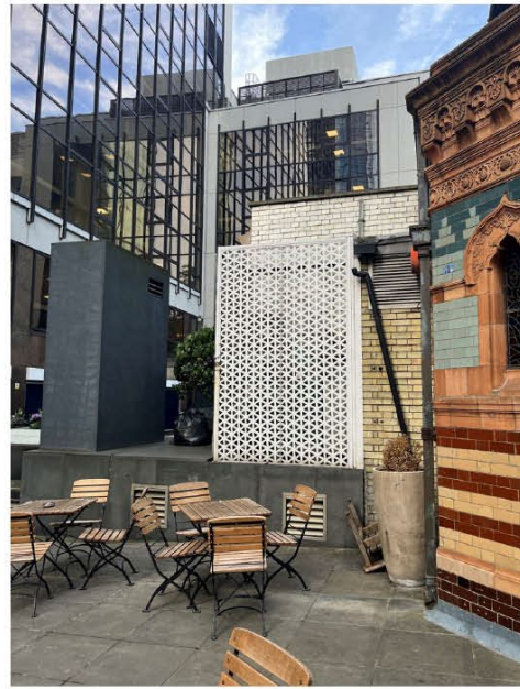
Figure 4 - View of 55 Old Broad Street and the Bath House from rear of existing Public House facing west.
