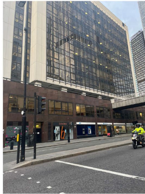
Figure 12 - View of 55 Old Broad Street from Wormwood Street facing north-east.
