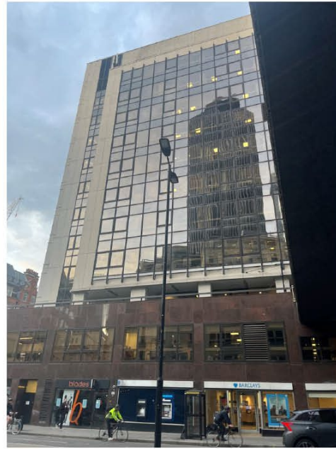
Figure 14 - View of 55 Old Broad Street from Wormwood Street facing north.
