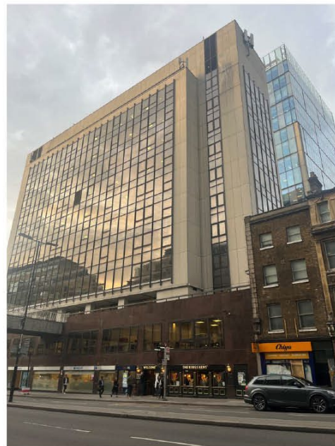
Figure 16 - View of 55 Old Broad Street from Wormwood Street facing north-west.
